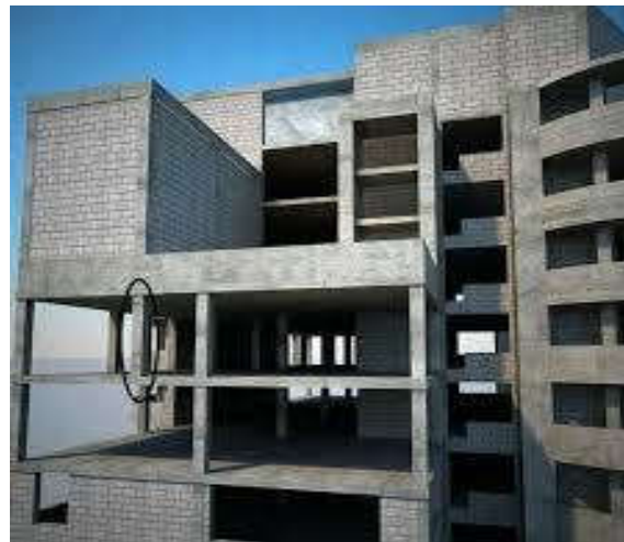
Fig.2 Typical Example of floating column
